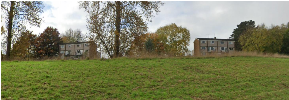
Photograph 4 – Four-Storey Apartment Blocks Overlooking Gadebridge Park
